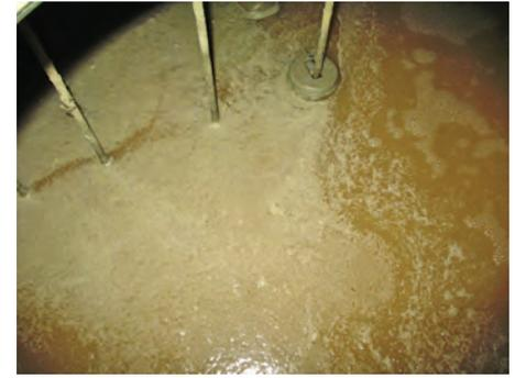
**Figure 3** — Any place where water has quiet dwell time, particularly dark spaces, such as pits, collection bags, trenches, tanks and recycling systems of all types can develop bacteria problems. The warmer and the darker the place, the higher the potential for problems.
